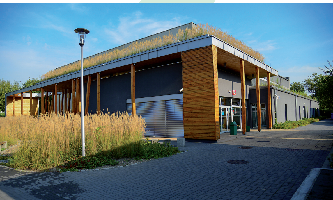
Passive design sports hall of the University of Agriculture in Krakow. Photo: A. Mróz
