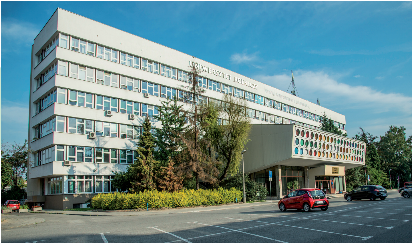
Building at al. 29 Listopada 54. Seat of the Faculty of Biotechnology and Horticulture. Photo: G. Wojcieszek
