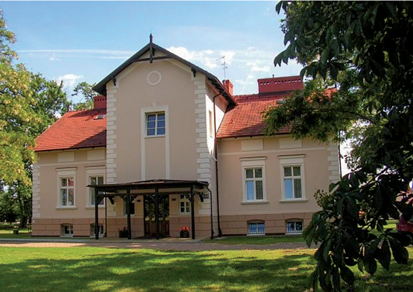
URK manor house in Mydlniki. Photo: URK Archive
