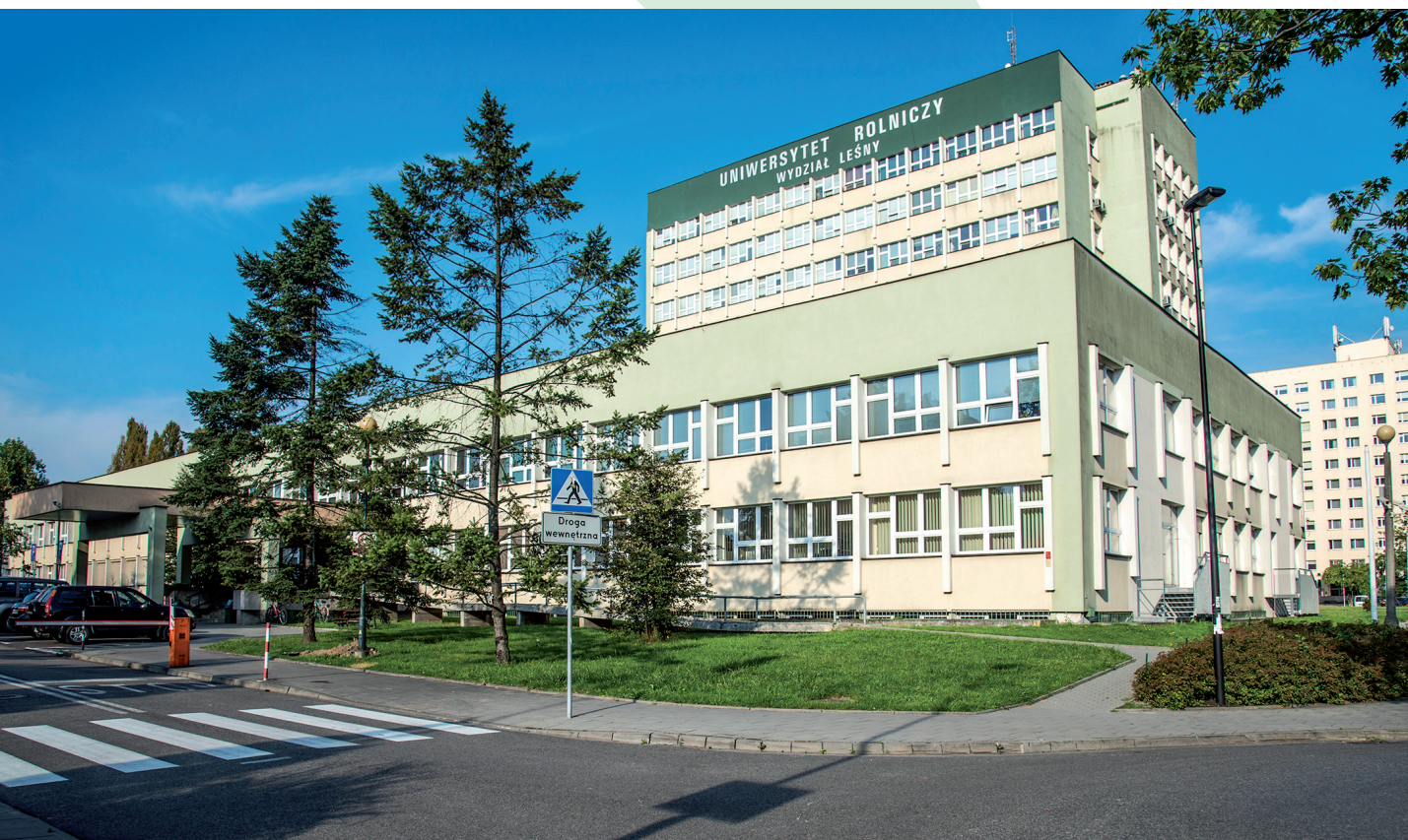
Building at al. 29 Listopada 46. Seat of the Faculty of Forestry. Photo: G. Wojcieszek
